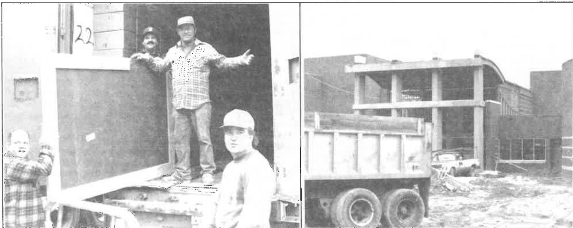
UNLOADING SUPPLIES are members of Laborers Local 543 of Huntington at Cabell Midland High School (right photo) at Ona now under construction. In the left photo are (from left) Rick Parsons, William Brammer, an unidentified employee of L&L Installation, and Steve Fulks. The project is financed with $5.8 million of West Virginia School Building Authority money and is being built around the existing Ona Middle School. It's been under construction since June, 1992, and is projected to be finished in time for the 94-95 school year. The new school will combine the students of Ona and Barboursville High Schools with an estimated enrollment of 2,200.
